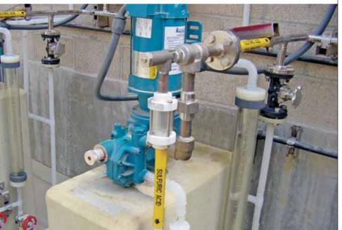
Sulfuric acid is one of the more challenging acids to pump, but some metering pumps are designed to handle this dangerous liquid.
