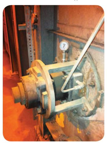
An Air Mizer seal permanently eliminates ash slurry from leaking out of a coal-fired boiler ash conveyor.
