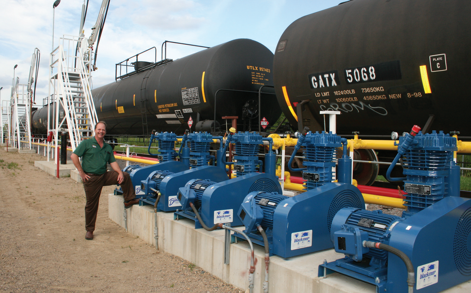
Pat Wenner, vice president of the Rockville Propane Terminal, has taken advantage of significant shifts in the propane supply and distribution market in Minnesota using reciprocating gas compressors.
