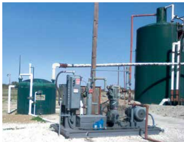
Oil-free reciprocating gas compressors help oil and gas producers and handlers meet the Quad O requirements.
