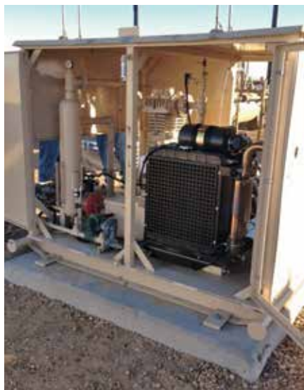
A vapor-recovery unit featuring an oil-free reciprocating gas compressor is a reliable way to control the amount of vapors that are lost to the atmosphere at a crude oil tank battery.
