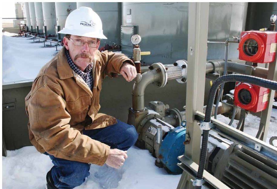
As part of his responsibilities, Tom Roberts, field supervisor for Pelican Gathering Systems, monitors the Pelican pipeline system, which utilizes pumps to introduce the oil and natural gas into the pipeline at the wellhead, transfer it through a series of switching locations along the pipeline and then deliver it to the storage tanks.
