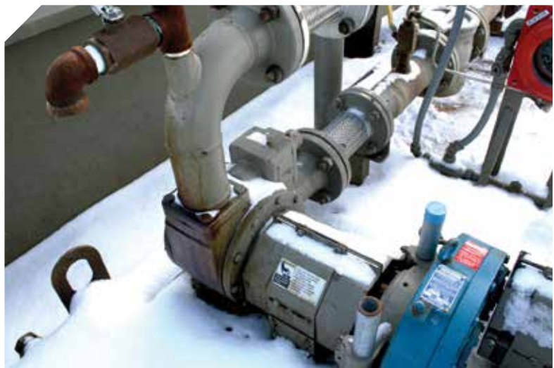
Image 1. These pumps can handle the harsh operating conditions found in the Bakken, where temperatures can reach -50 F. (Images courtesy of Blackmer)
