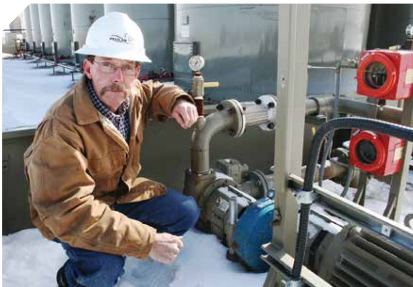
Image 3. As part of his responsibilities, Tom Roberts, field supervisor for Pelican Gathering Systems, monitors the Pelican pipeline system, which uses pumps to introduce the oil and natural gas into the pipeline at the wellhead, transfer it through a series of switching locations along the pipeline and then deliver it to the storage tanks.
