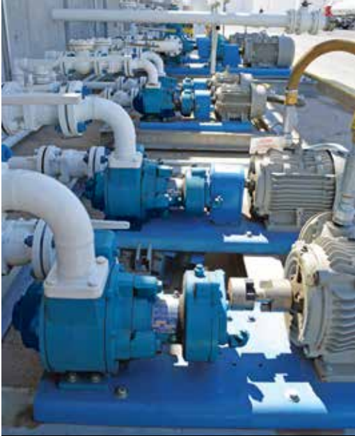
Image 3. In sliding vane pumps, the vanes form pumping chambers that transfer fluid as the rotor turns.
