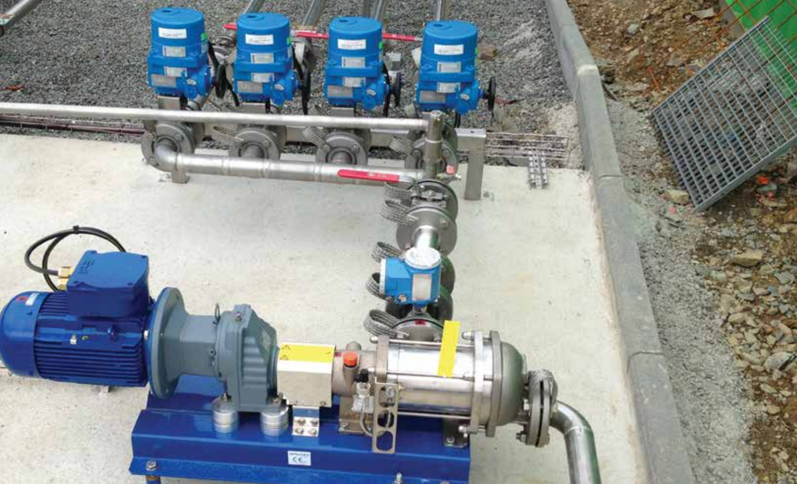
Image 1. Eccentric disc pumps can reliably transfer commodities as diverse as ethanol, pharmaceuticals, isocyanates and paints. (Courtesy of Mouvex)
