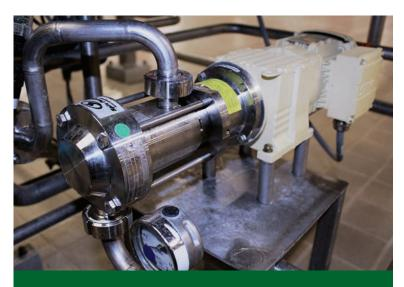
The Mouvex® SLS Series is the pump of choice for the 's-Hertogenbosch brewery because they are sealless, highly reliable, volumetrically consistent, easy to clean and require low maintenance.
