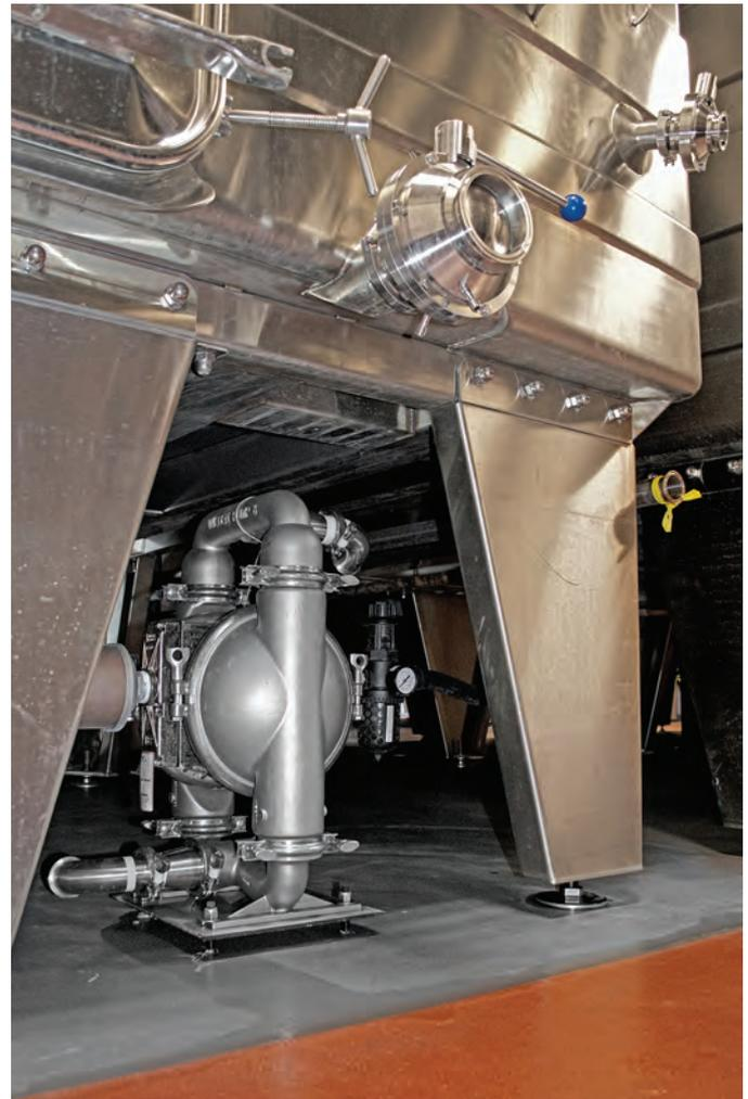
Wilden® PS8 Saniflo™ FDA pumps equipped with the Pro-Flo® SHIFT Air Distribution System (ADS) and Full-Stroke Integral Piston Diaphragm (FSIPD) provide maximum cleanability and energy savings for cap irrigation at Rodney Strong Vineyards.
