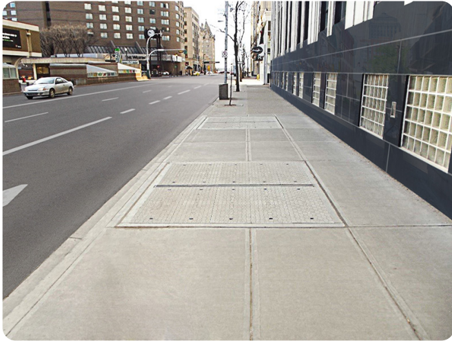
Finished cover installation in Edmonton
