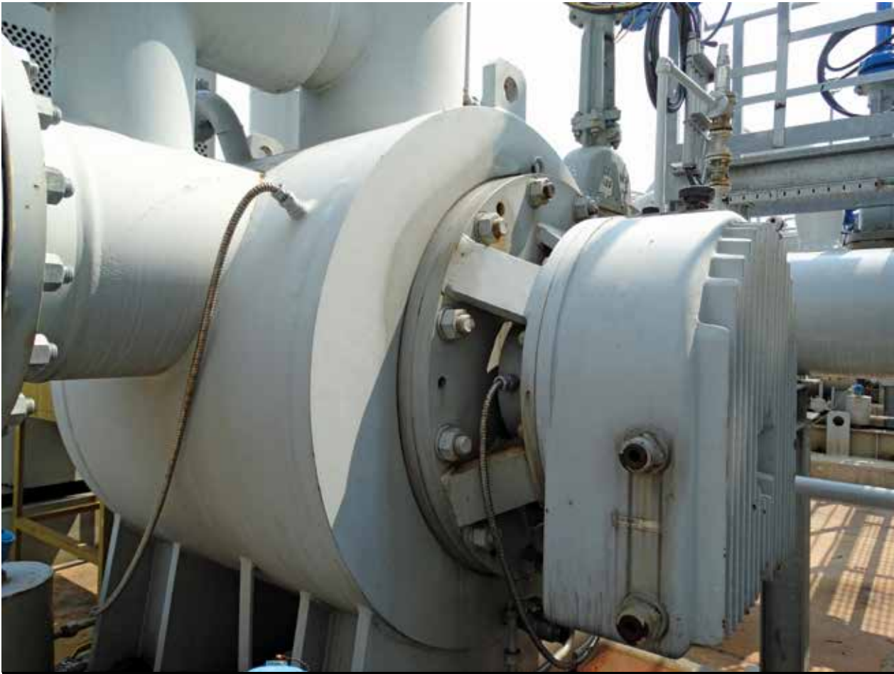
Image 2. These triple screw pumps are made to handle clean lubricating fluids without solid content across a wide range of viscosities, temperatures and pressures. This method of operation delivers smooth, constant product flow with low noise and high levels of energy efficiency.
