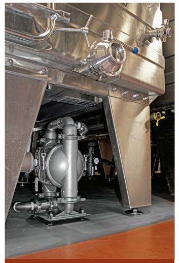
Wilden<sup>®</sup> PS8 Saniflo<sup>™</sup> FDA pumps equipped with the Pro-Flo<sup>®</sup> SHIFT Air Distribution System (ADS) and Full-Stroke Integral Piston Diaphragm (FSIPD) provide maximum cleanability and energy savings for cap irrigation at Rodney Strong Vineyards.
